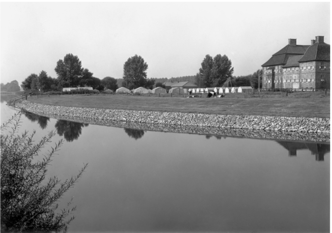
At the beginning of September 1969 the bank had been sloped back and reinforced with a stone rip rap embankment.
