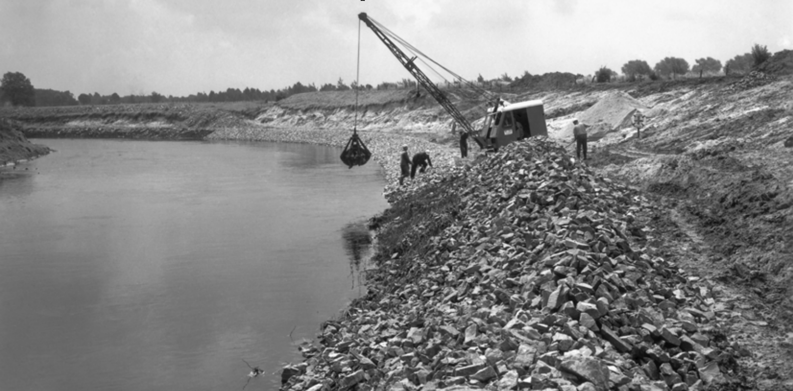
A picture from the 1960s: A construction crew of the Lippeverband securing an undercut bank.
