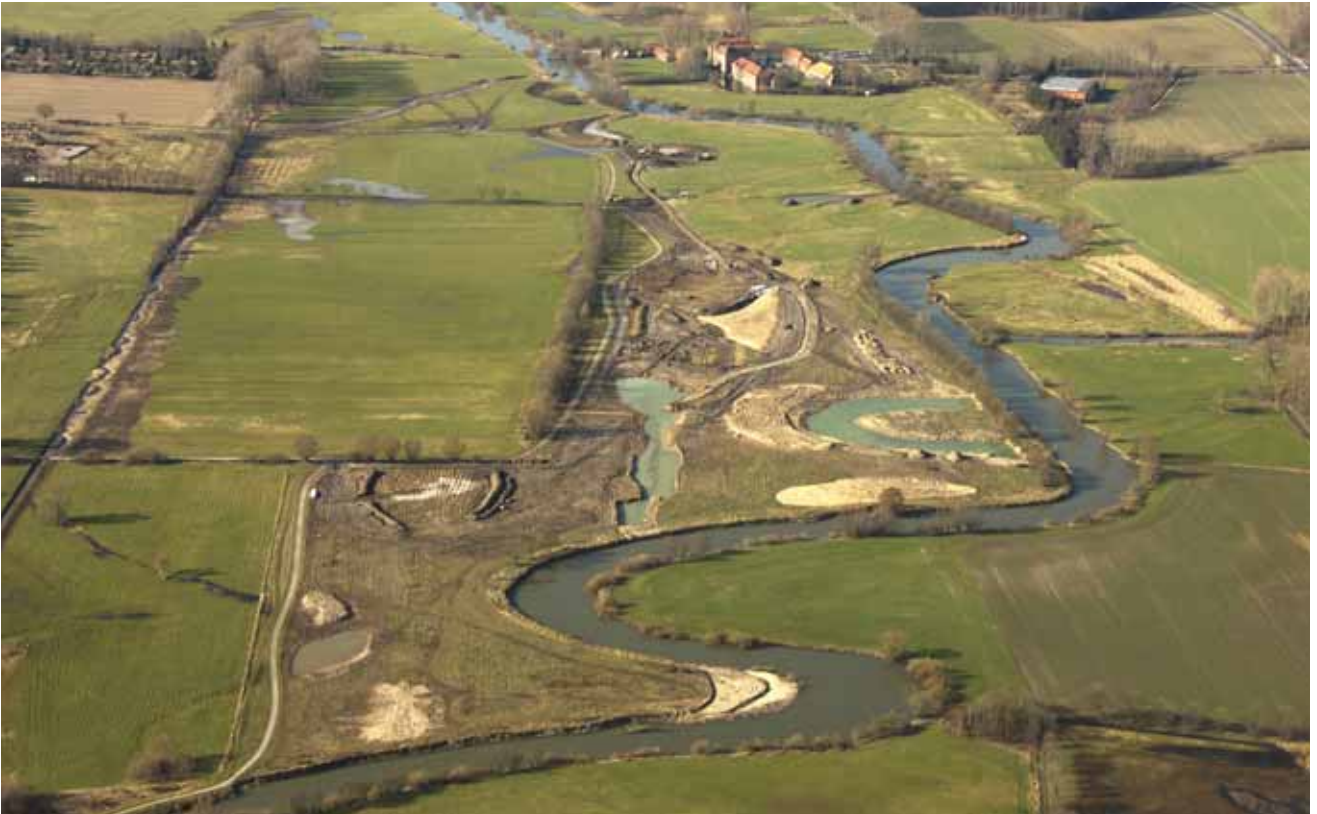
Block C as a construction site: The path has already been relocated into the meadows at the centre of the floodplain area, the river banks have been restored to a natural state and the Lippe has been widened. In the centre of the photo, construction vehicles are modelling new areas for standing water and constructing the observation hill.
