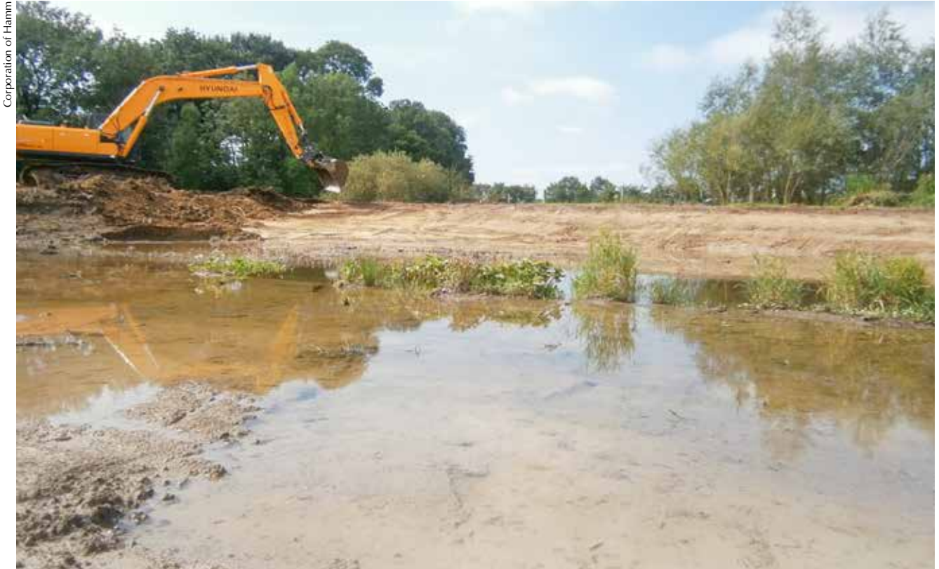
Excavator digging a flood channel.
